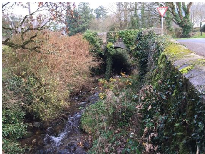
Plate 10-1 BH 1, facing northeast
